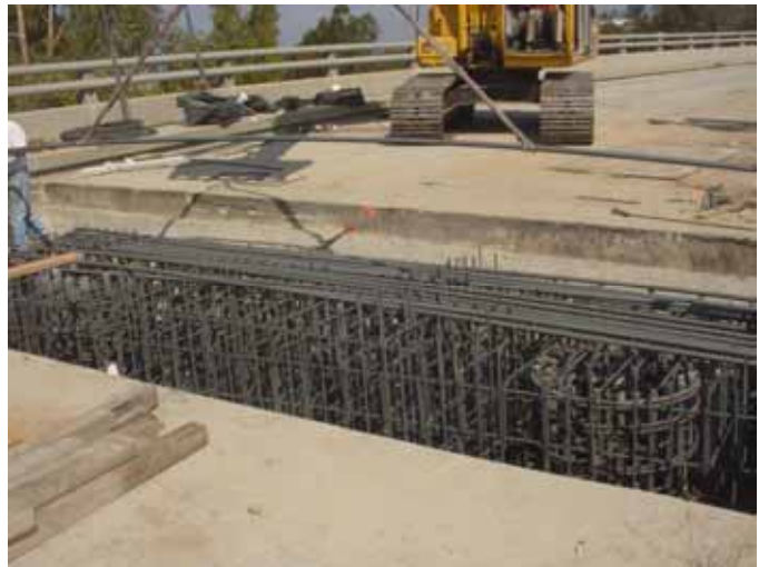
Reinforced Concrete Pile Cap
