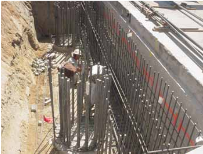
Drilled Cast in Place Pilings
