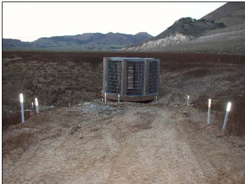
Twitchell Emergency Sediment Removal Project Completion
