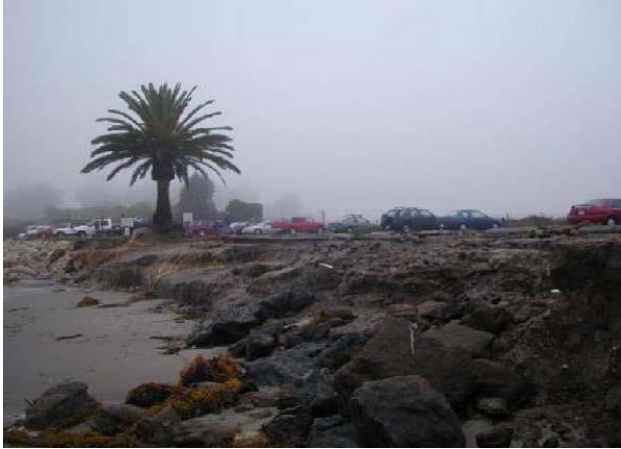
Storm wave action – 34 parking spaces lost
