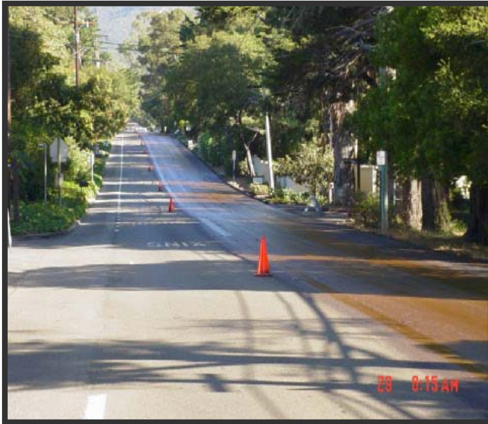
Figure 1: Fog seal applied to one lane.
