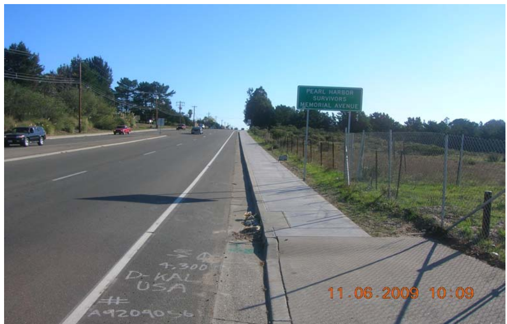
New Sidewalk on Clark Avenue in Orcutt
