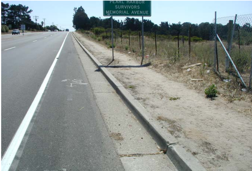
Clark Avenue in Orcutt prior to Construction
