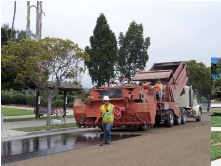
Applying Scrub Seal
