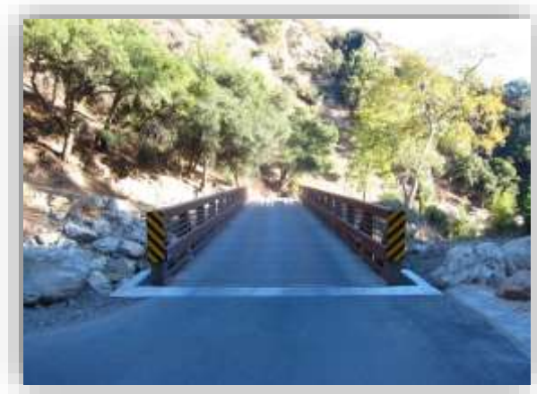
Existing Condition with Temporary Bridge, December 2020 (view east)
