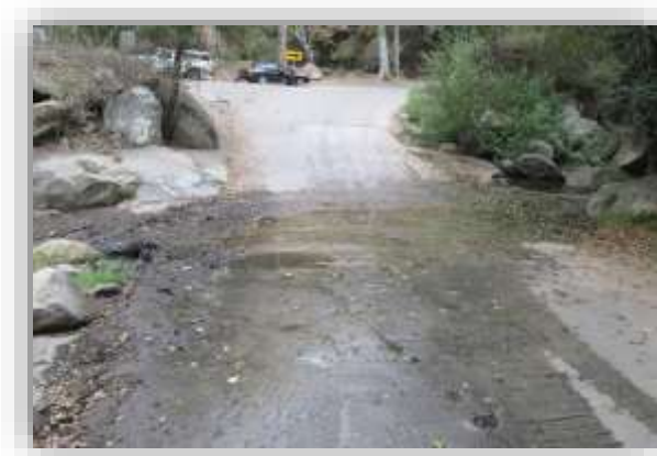
Low Water Crossing Pre-TFDFI (view west), September 2016
