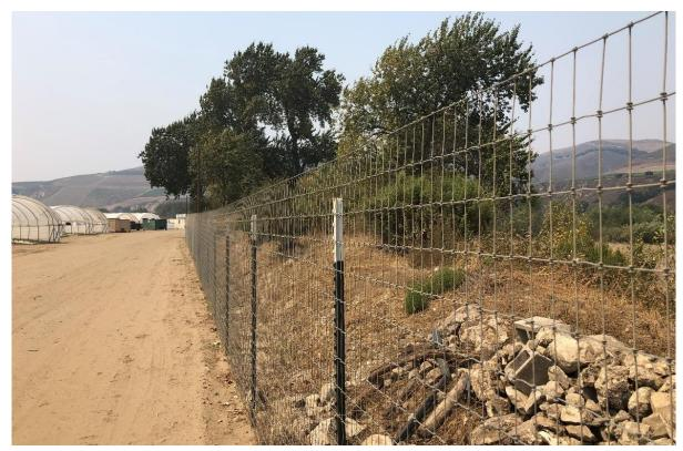
**Photograph 10.** Perimeter fence along northeast portion of proejct area seperating cannabis area from riparian vegetation. Note six-ft-tall fence and natural berm (aspect west; August 19, 2020)
