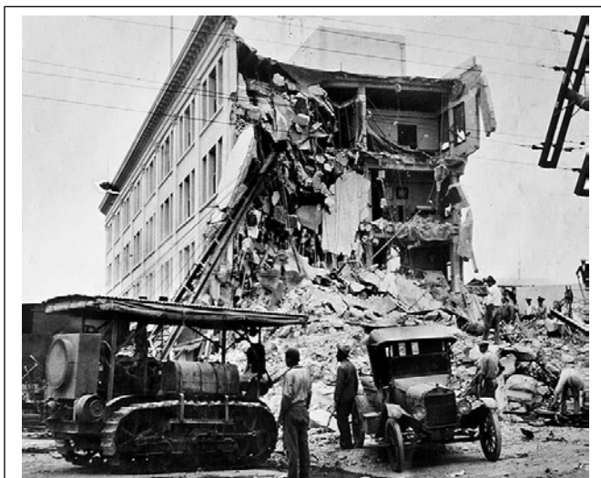
Damage from the 1925 Santa Barbara earthquake
