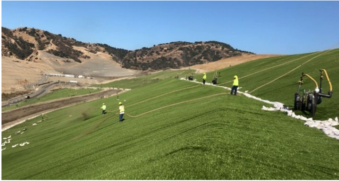
Installation crew spraying infill sand into the newly installed closure turf.
