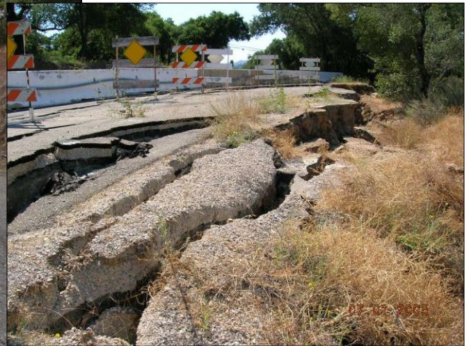
Failed Roadway on Paradise Road at MP 2.5
