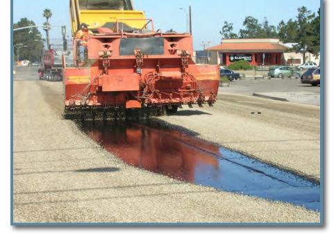
cost of a traditional overlay. It is typically overlaid with a micro surface for ride quality and to add further life to the pavement
