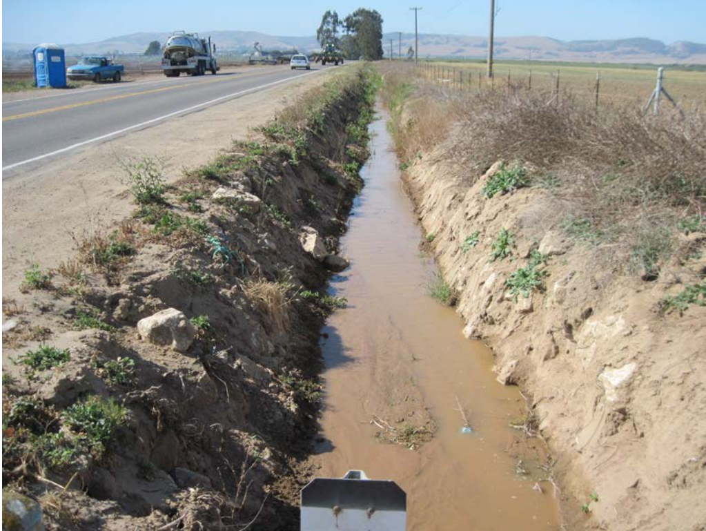
Photo 3. View of the agricultural ditch along the east boundary of the project site. Photo was taken in the northeast corner of the site facing south.
