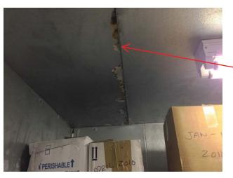
Walk-In Cooler Ceiling Corrosion.
