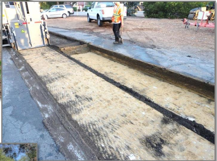
*Removing failed areas on Las Palmas Drive*
