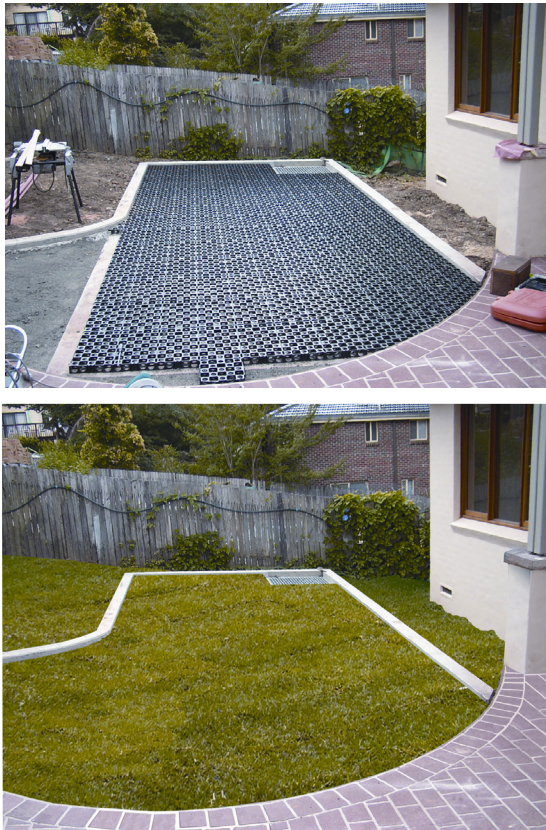
Figure 3.9 – Grasscell Used to Manage Stormwater Runoff
