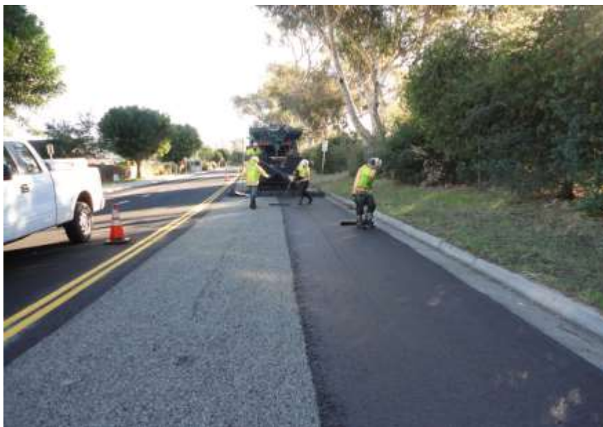
Placing Micro-Surfacing on Calle Real
