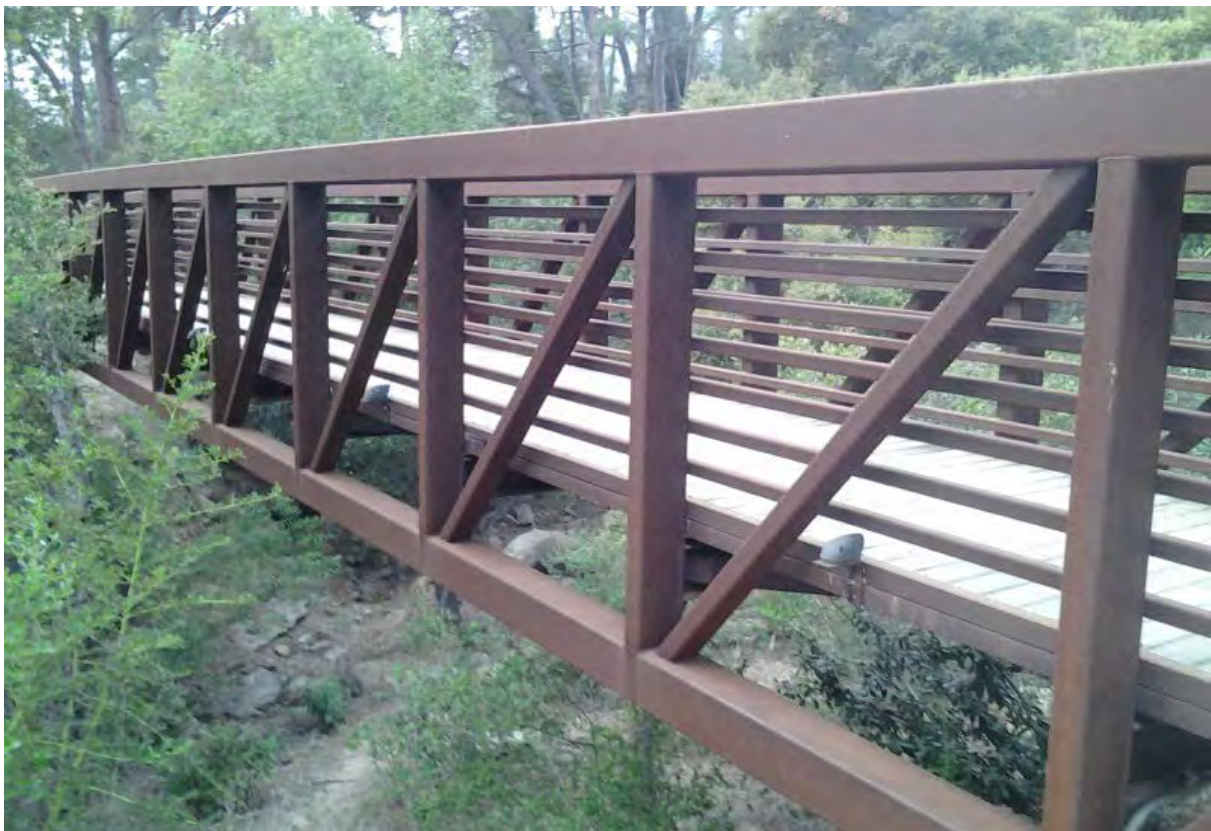
Westmont College Ped Bridge (129' span, 7' truss height)
