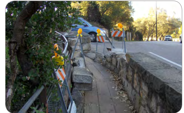
ACCIDENT DAMAGE TO MISSION CREEK BRIDGE
