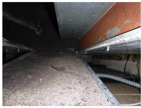
This shows the extremely heavy accumulation of dirt in one of the room terminal units.
