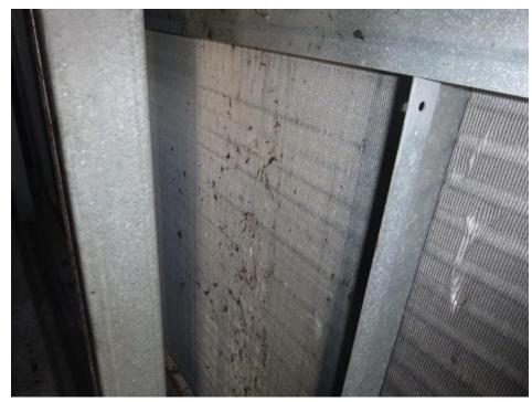
The cooling coils are also getting dirty, which reduces efficiency and increases energy costs.
