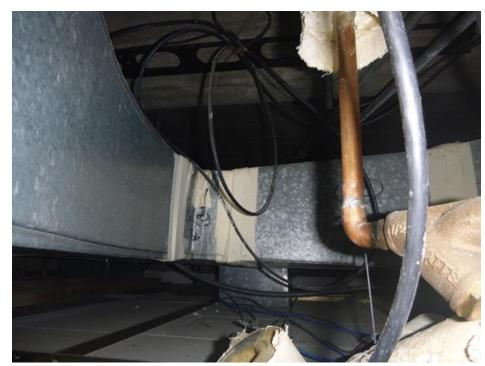
The ducts on the roof and most of the ductwork inside the building is internally insulated, as shown here.
