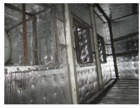
This photograph from one of our recent projects shows a similar air handler after we cleaned and sanitized, and installed new Reflectix nonfiberglass insulation. This is a representative example of our work.
