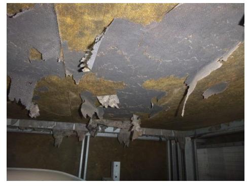
The interior walls of the air handlers are lined with fiberglass insulation. This fiberglass liner is deteriorating, which also needs to be addressed as part of our scope of work.
