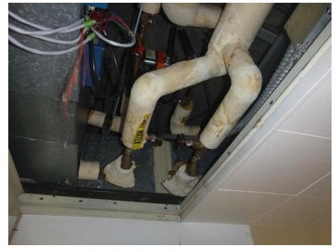
We will thoroughly clean the interior of the room terminal units, including the reheat coils.
