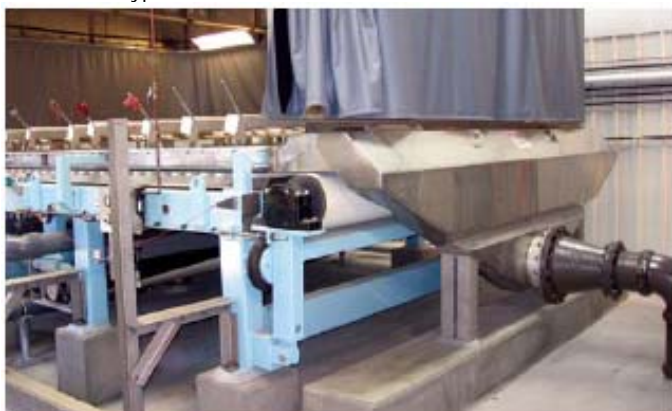
FIGURE 3-9 Picture of a Typical GBT
