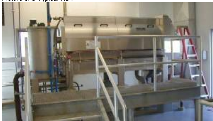
FIGURE 3-11 Picture of a Typical RDT
