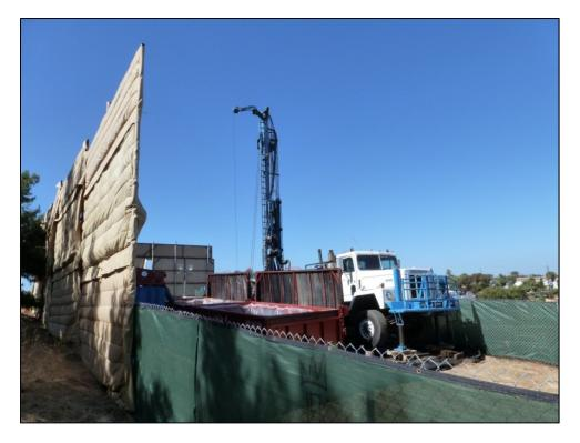
Figure 17 – Sample Temporary Construction Noise Barrier (URS, 2012)
