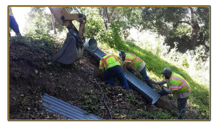
When water collects on or adjacent the roadway, it permeates the asphalt and/or penetrates into the subgrade and stresses the pavement. Cracking develops over time, eventually causing the pavement to disintegrate. Routine culvert drainage maintenance helps prevent this type of water damage on the roadways. The faster water drains from the roadway, the better it is for the life of the pavement.
