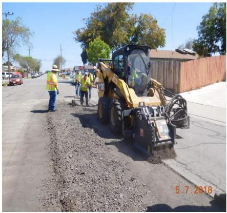
Surface preparation as well as maintenance includes repair and maintenance of existing pavement surfaces, as well as surface treatment preparations for projects. These activities include, but are not limited to: skin patching, pothole patching, crack sealing, and fog sealing. County crews perform these corrective procedures to re-pair potholes, fill cracks, and level asphalt settlement in both rural and urban areas.
