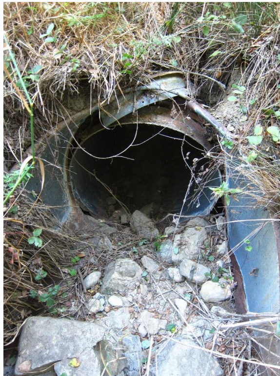
Jalama Road Culvert Inlet
