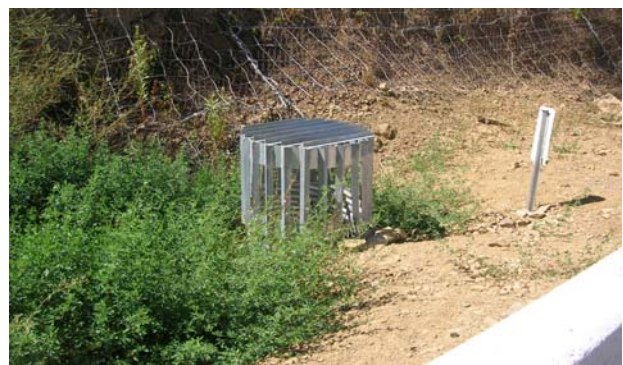
Stagecoach Rd MP 3.5 Inlet Debris Rack Riser
