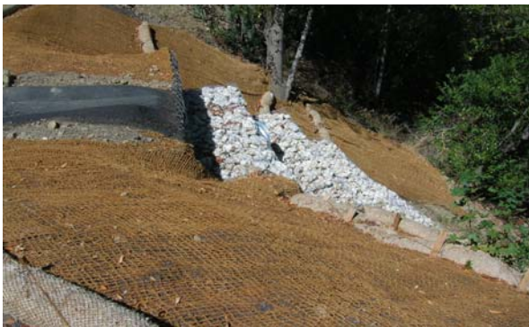
Stagecoach Rd MP 3.5 Gabion Outlet Drainage
