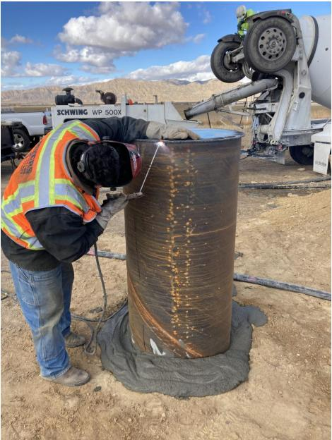
Welding 32'' steel cap on top of 30'' steel casing SBCPHD Well Permit WP#0004497 Suarez Property, 2225 Foothill Road, New Cuyama, California, APN 149-160-033
