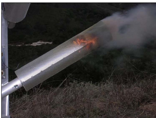
Figure 4 Flare burning inside spark arrester
